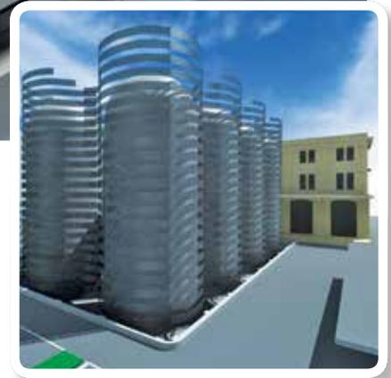
The essential function of the accumulation system is the storage of the thermal energy produced by thermoelectric power plant in cogenerations overnight, when the heat demand for heat is lower and its use during the hours of maximum load of the district heating system, minimizing the use of the integration boilers.
